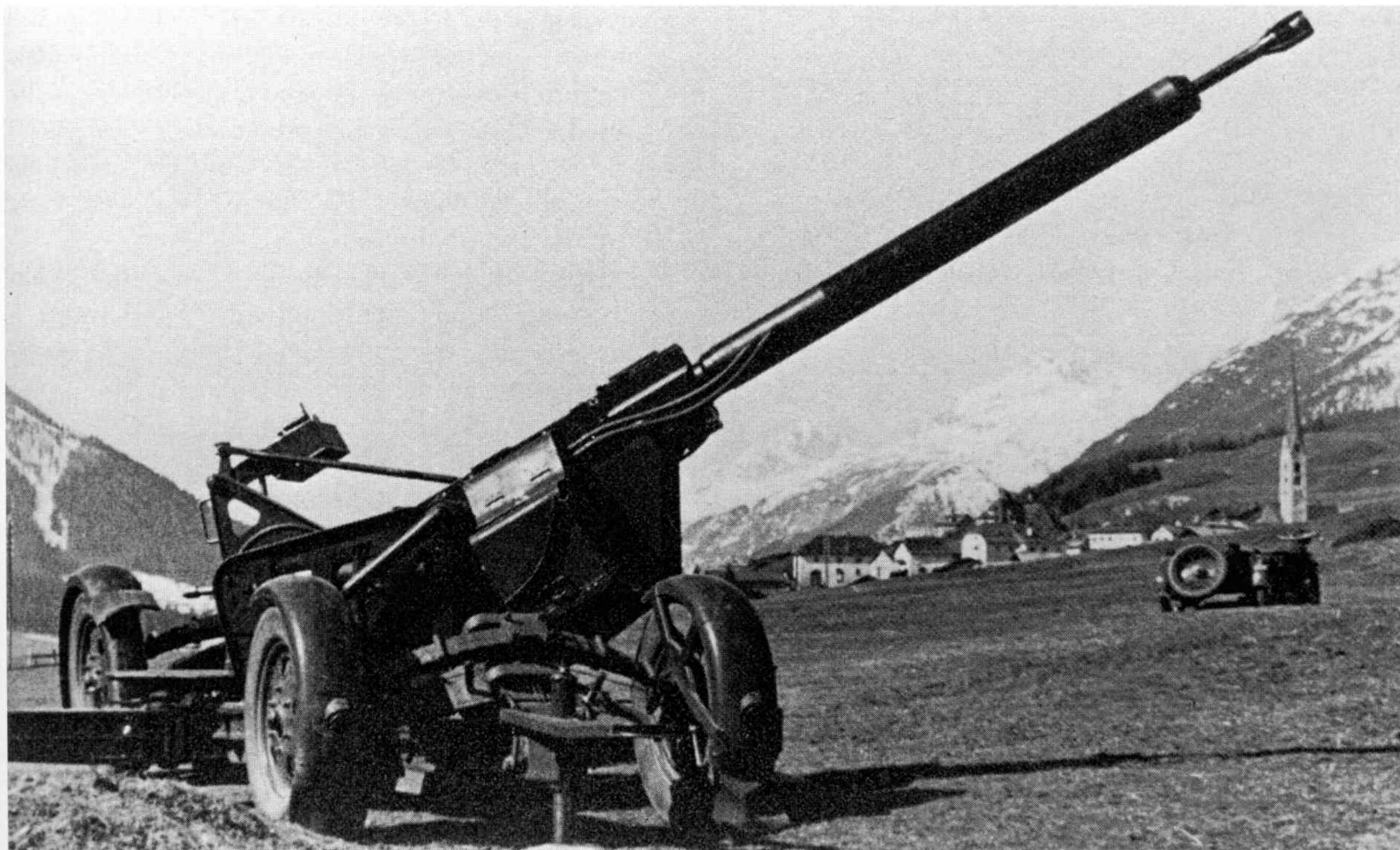
Swiss 34mm Flab. Kan. 38: note water-cooled barrel (Courtesy: Verlag Stocker-Schmid, Dietikon-Zurich)
