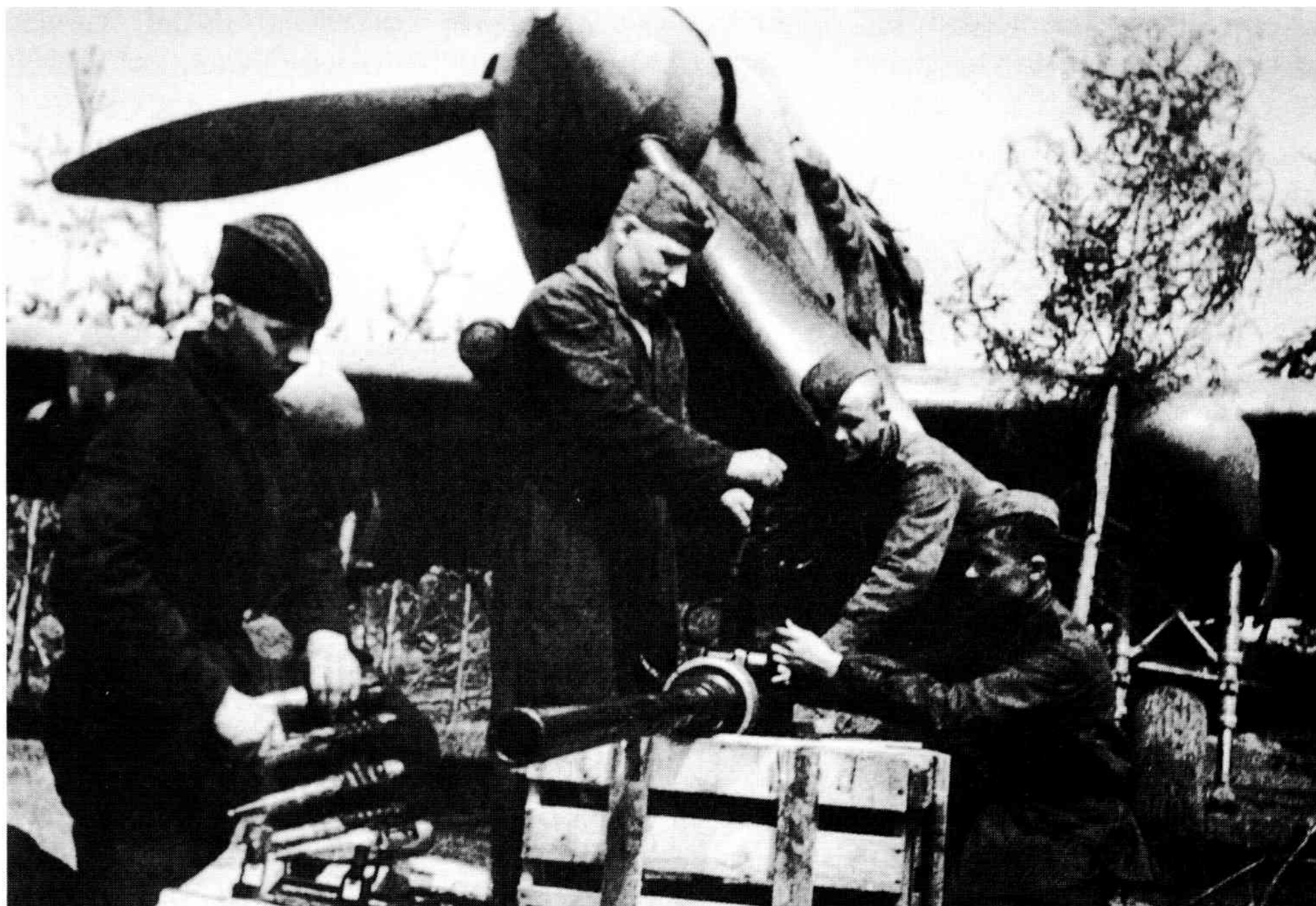
NS-37 gun and ammunition by its Ilyushin Il-2 3M Shturmovik aircraft
